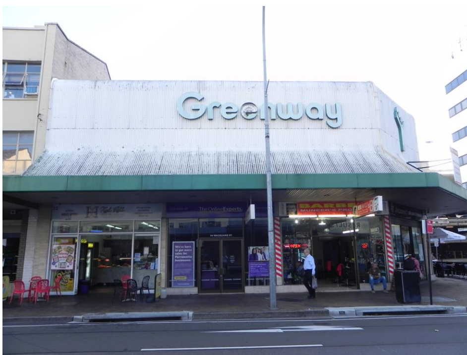
Figure 3 – The 'Greenway Plaza' as viewed from Macquarie Street Source: JBA
