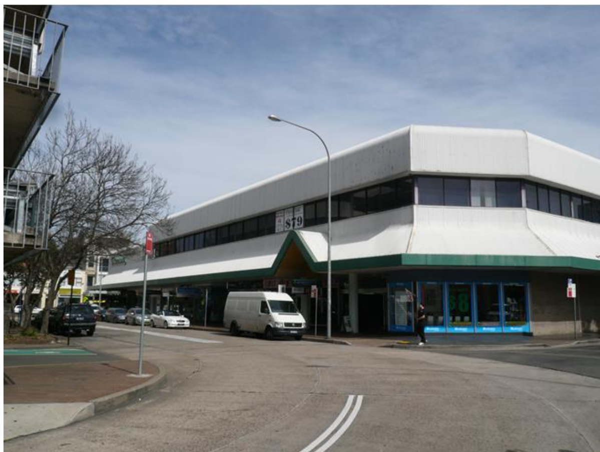
Figure 6 – The Greenway Plaza, as viewed from Horwood Place Source: JBA
