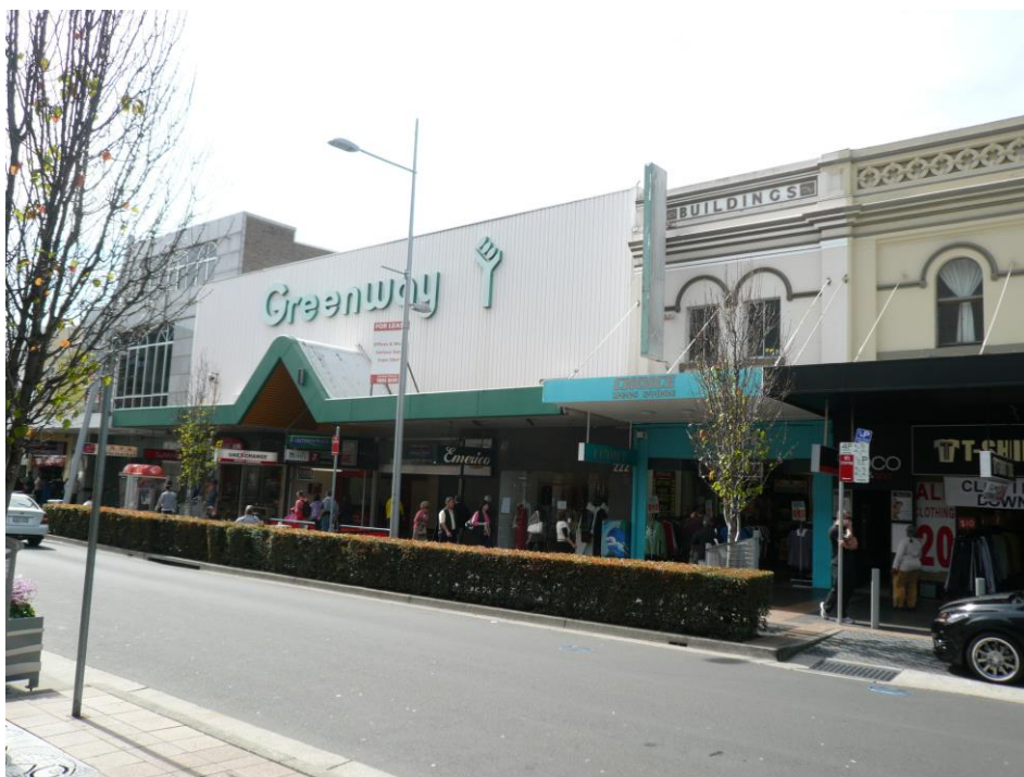
Figure 5 – 220 and 230 Church Street, as viewed from Church Street Source: JBA
